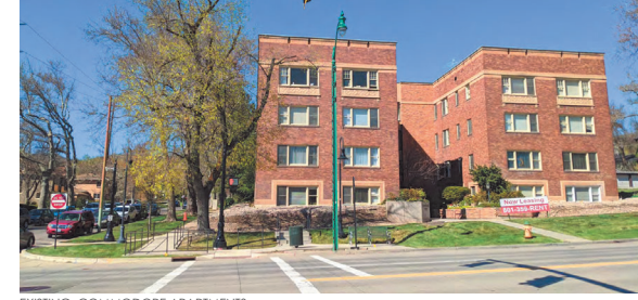
EXISTING: COMMODORE APARTMENTS
