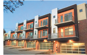
ALMOND STREET PROJECT BY GARRETT HOMES 275 N. WEST TEMPLE
