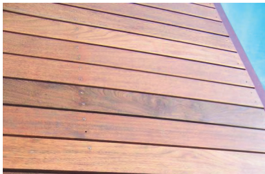
HORIZONTAL WOOD SIDING DETAIL
