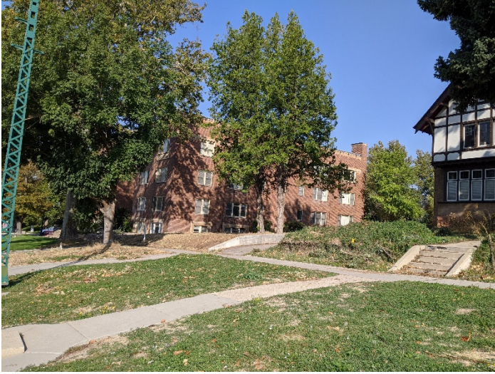
Figure 13 – Southeast view of the lot
