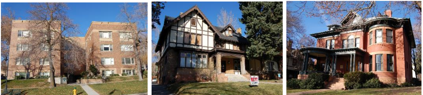
Figures 1, 2 and 3 – Structures located on the same block face as the subject property. The structures reflect different periods and styles and are considered contributing to the South Temple Historic District.
